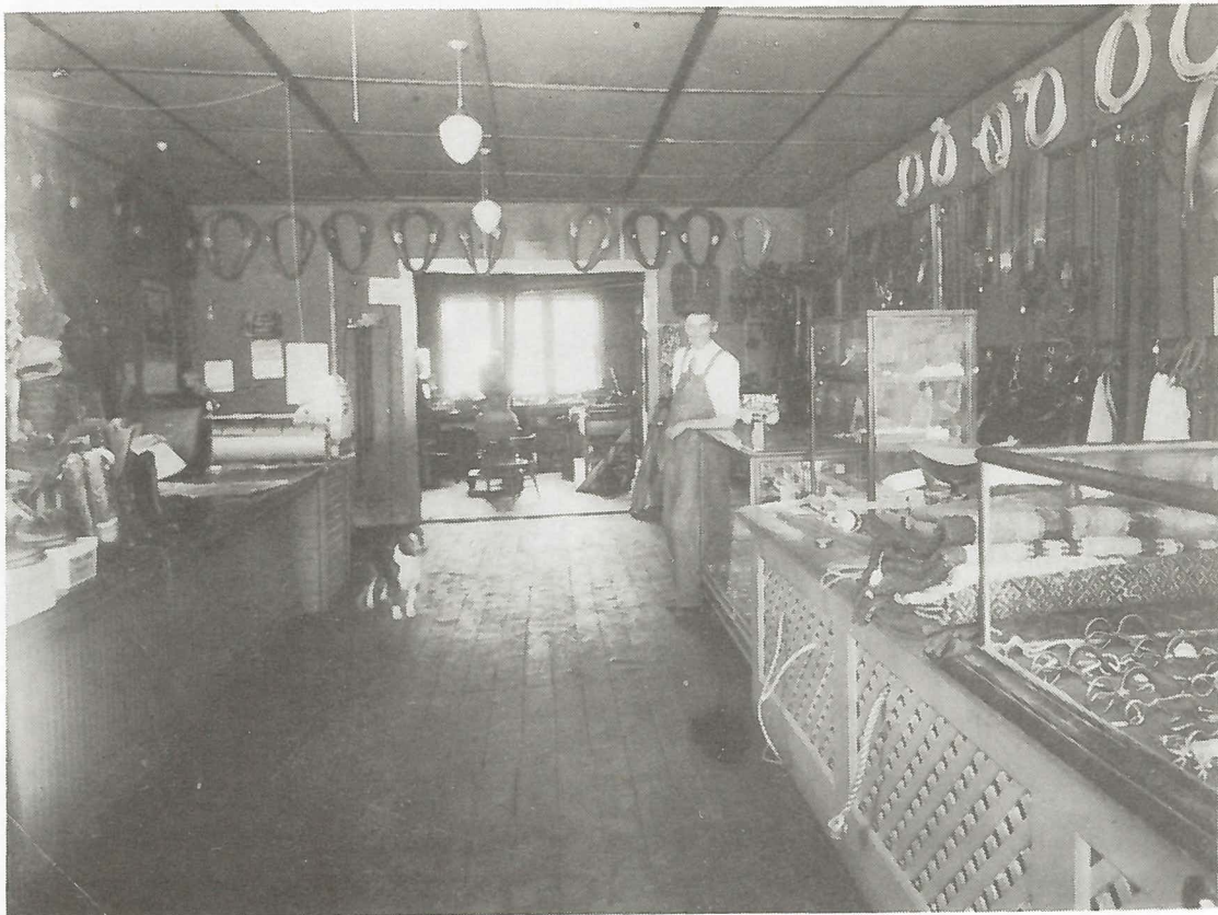
CHARLES HARWIG IN STORE AFTER REMODELING
